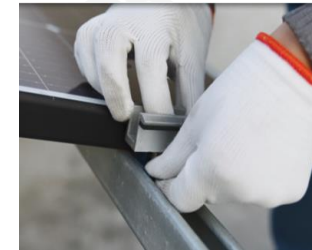
Fig. 4 & 5 – Installation of Full-Screen panels using mid/end clamps with rubber pad(s) attached
